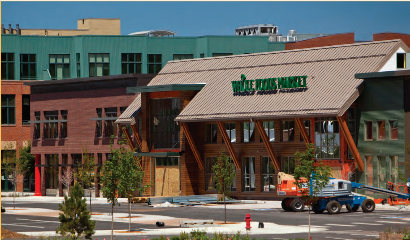
The new Whole Foods complex under construction at Willits Town Center. (Photograph from June 2012)
